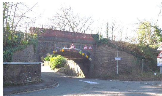
High St, Sandhurst low bridge (A231)
