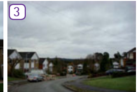
Mostly gable ends front onto street
