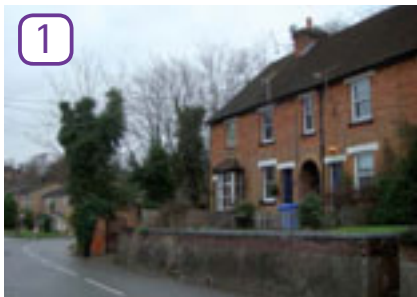
Retaining wall creates distinct boundary treatment
